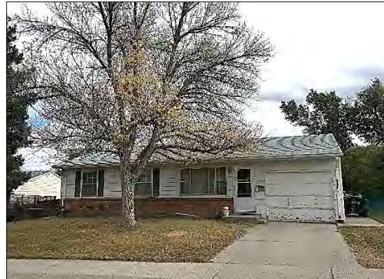
c1960 Ranch Style house, 2601 Navarre Rd.
