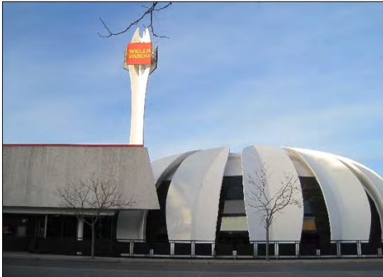
1964, Expressionist bank building, 234 East 1 st St.
