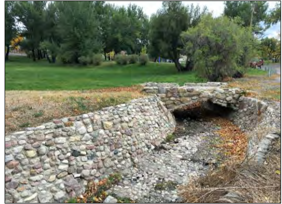
1930s Washington Park Grounds, 951 S. Jefferson St.
