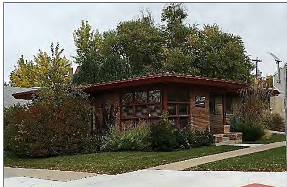
c1949 Contemporary Style office, 843 S. Center St.
